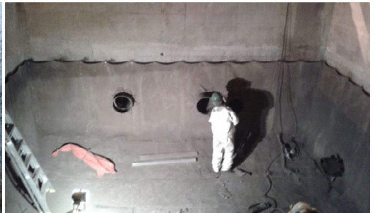
Completed installation (00:30 hrs)
