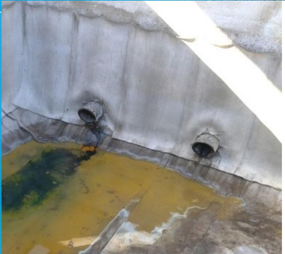
Completed lined acid tank 9 hours after hydration.
