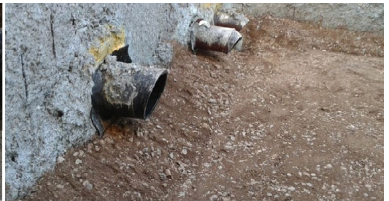
Recovering the tank ground level with graded earth
