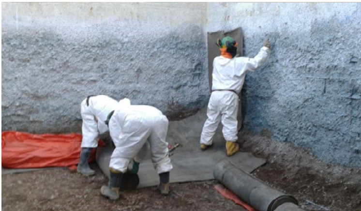
Start of CC installation (16:00hrs)
