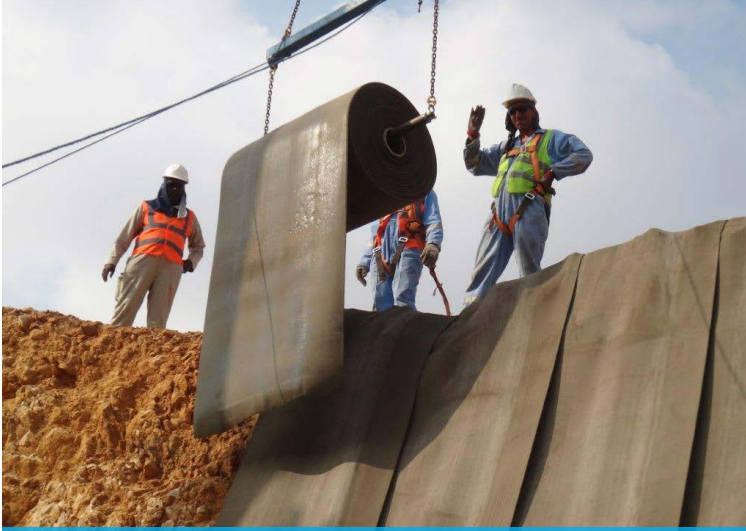
CC being lifted into position
