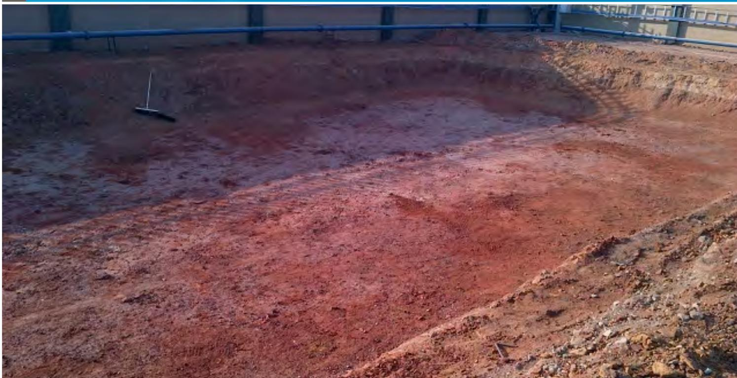
The dam site was excavated and cleared by an on-site team prior to installation of CC
