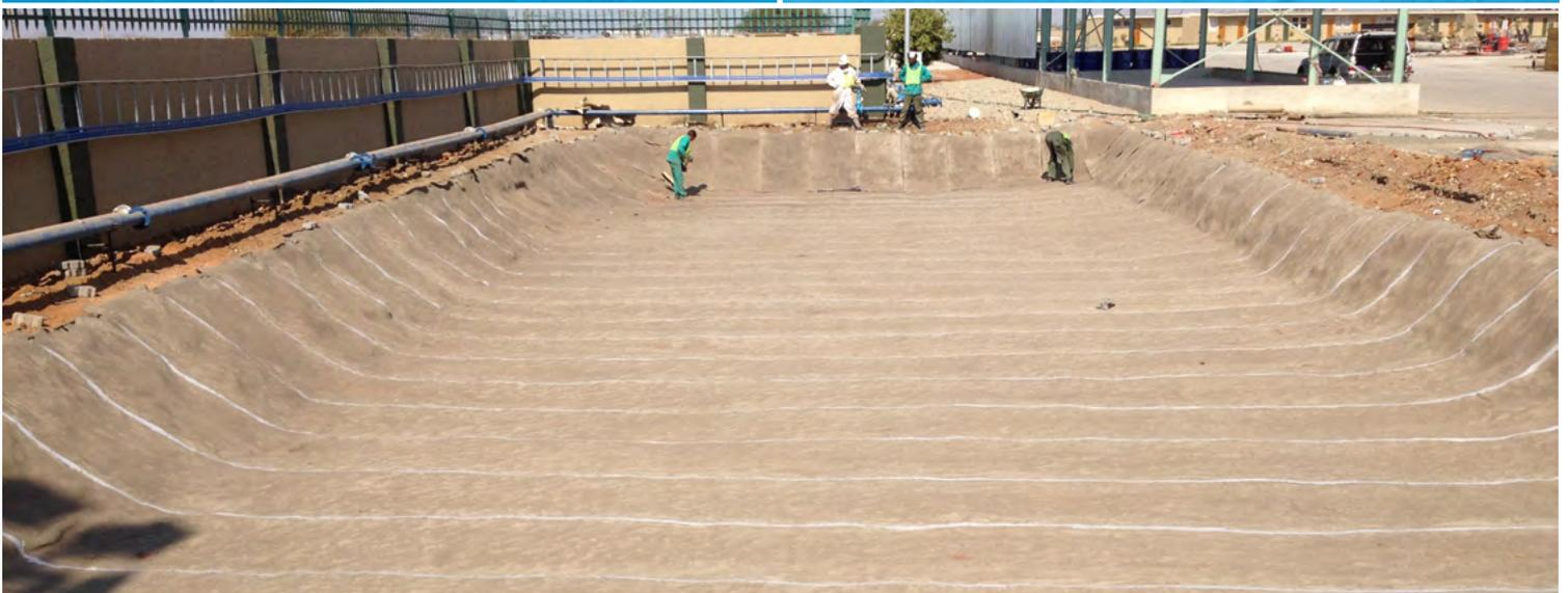
*A UV-resistant, waterproof sealant was used to seal the joints on the concrete side*
