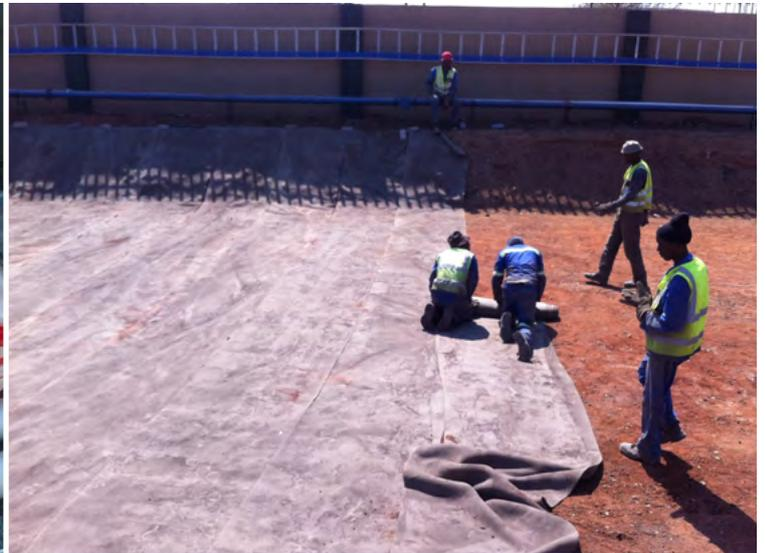
*Joints between layers of CC were sealed with a VHB tape underneath*
